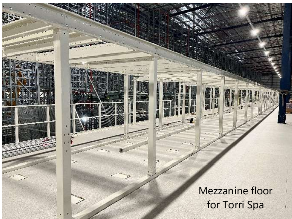
Mezzanine floor beams for Torri Spa under construction with a Witron sequencer beyond.
