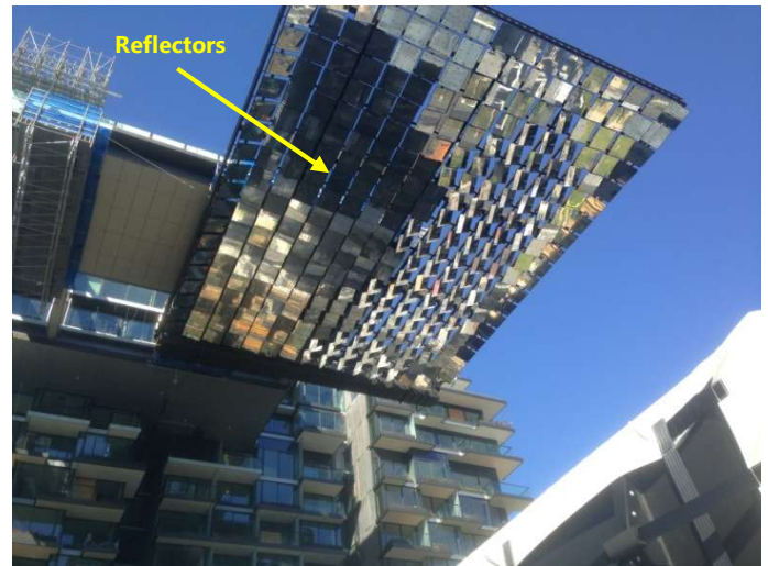
Upward view at the east tower cantilever supporting the reflectors.
